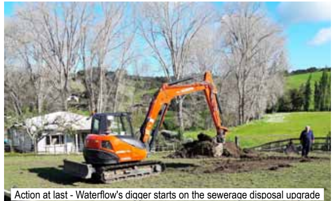
Action at last - Waterflow's digger starts on the sewerage disposal upgrade
